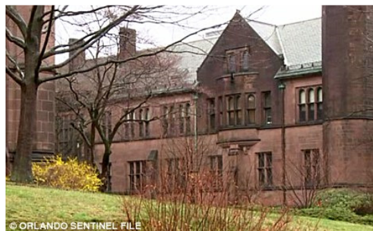
Death scene: Yale's Sterling Chemistry Laboratory where Michele died in the basement machine shop
