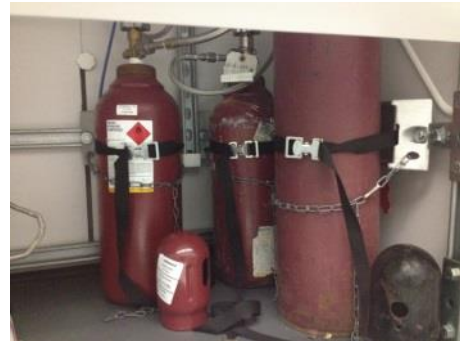
One chain for small cylinders. Straps for back-up
