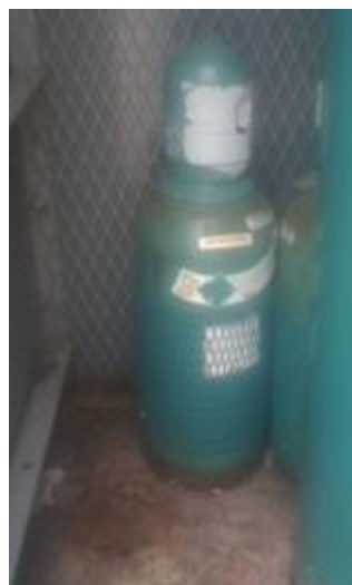
Figure 1: Small SF 6 cylinder last used 6 years prior, note rust creeping up from base of cylinder.
