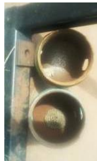
Figure 2: Both cylinder caps include wasp nests.
