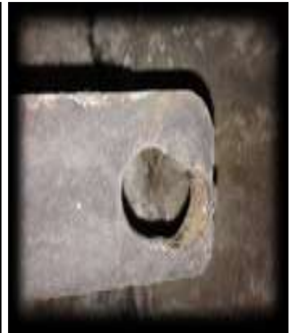
Figure 3. Damaged lifting eye
